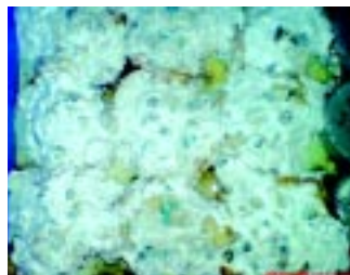
Damaged OPC Concrete under H 2 SO 4 Attack
