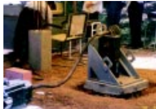
Dynamic Test on Pile
